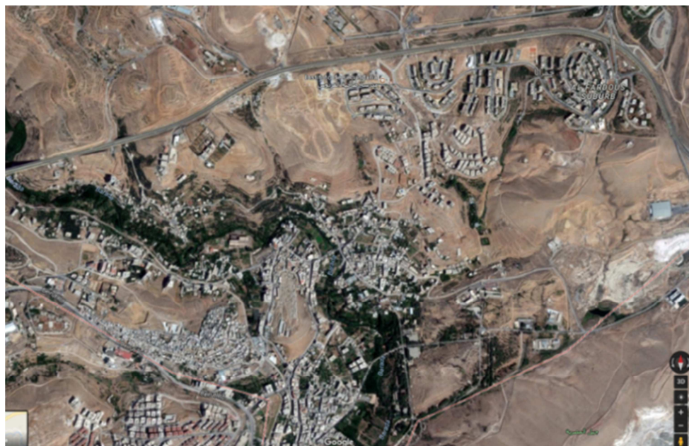
Figure A2. Al Hamah area, a river crosses the area.
